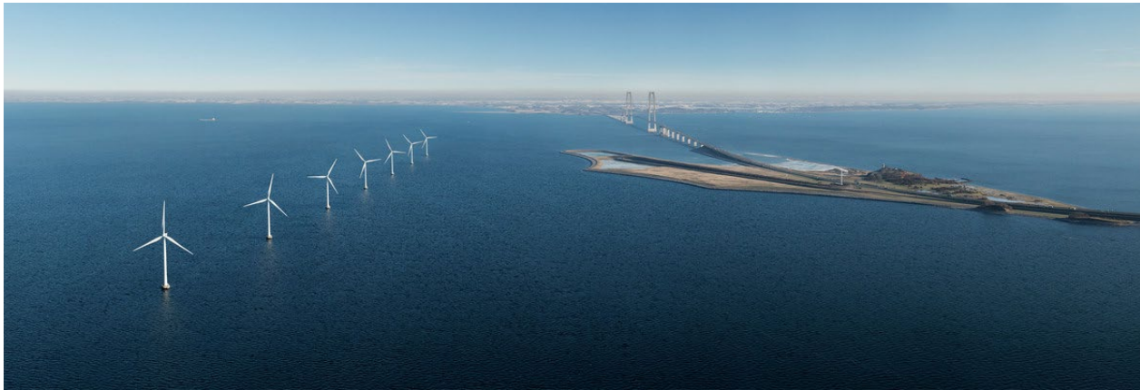
Credit: MHI Vestas Offshore Wind
